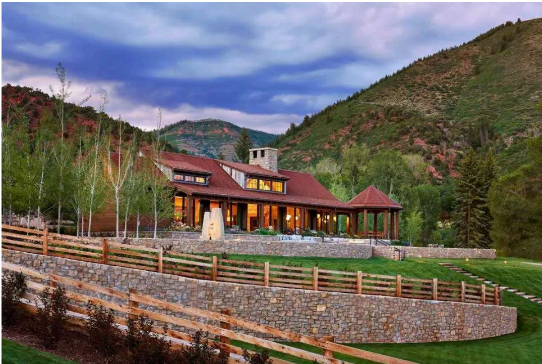
Ranch House at Aspen Valley Ranch. ASPEN VALLEY RANCH
