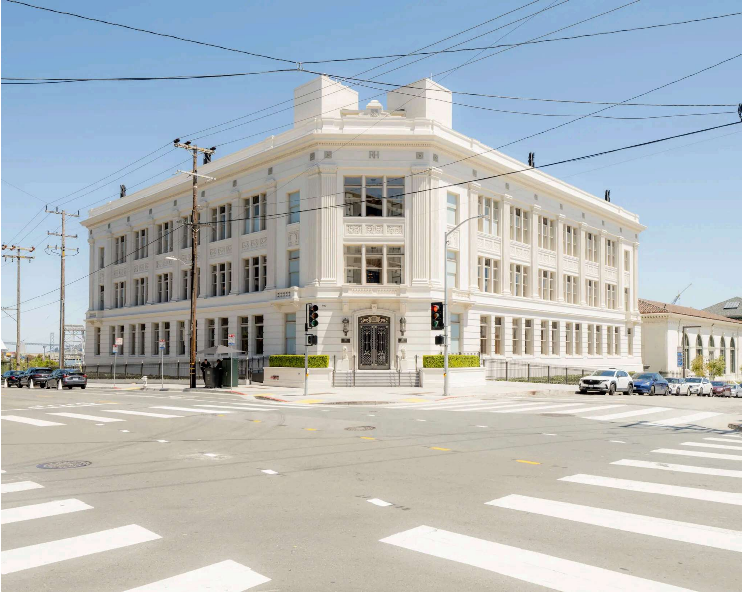
RH San Francisco, which includes retail and restaurants, occupies a former Bethlehem Steel building. Cayce Clifford for The New York Times
